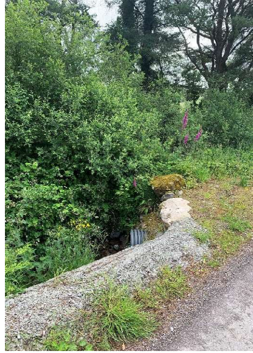
Image : 32 Storm water pipe crossing under road at this location.
