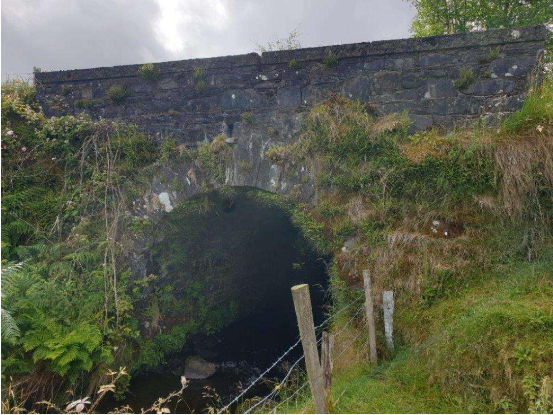
General view of the east elevation
