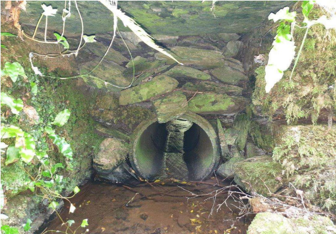
Repair to existing culvert with a 450mm concrete drainage pipe (south span).
