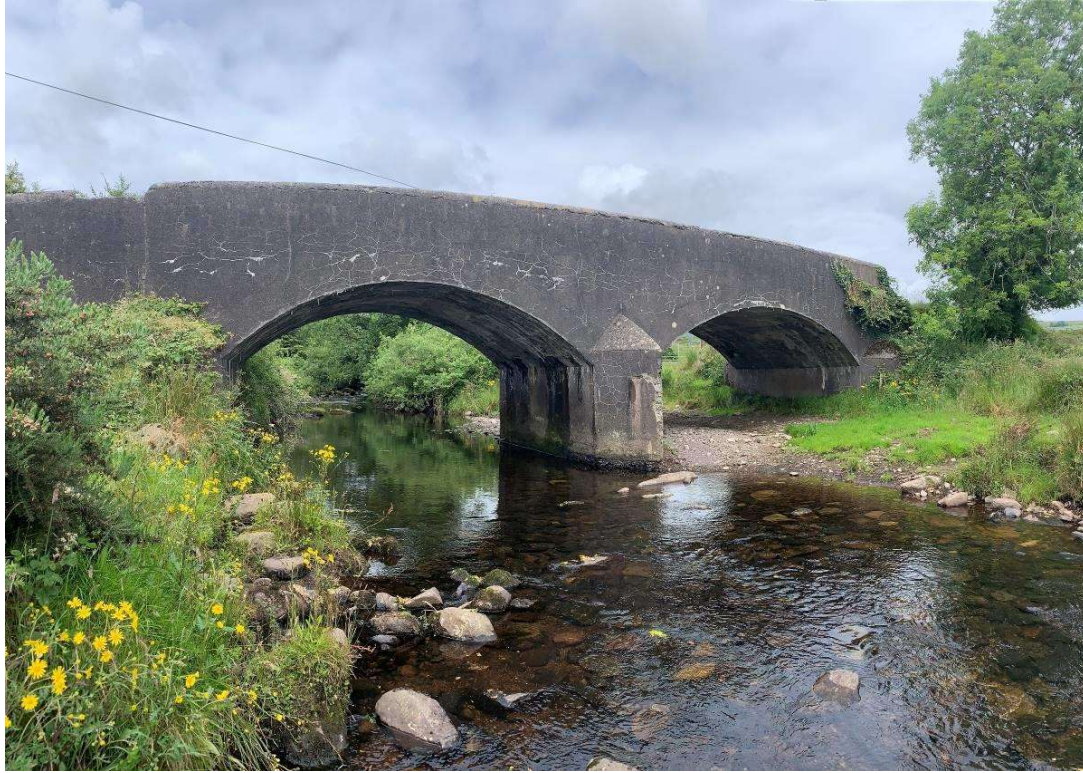
General view of bridge elevation - viewed from downstream.
