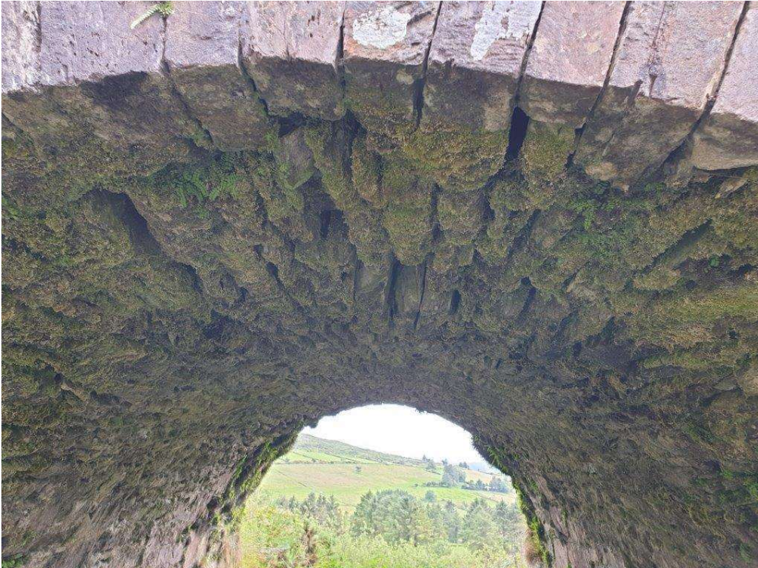
General view of the arch barrel from the north
