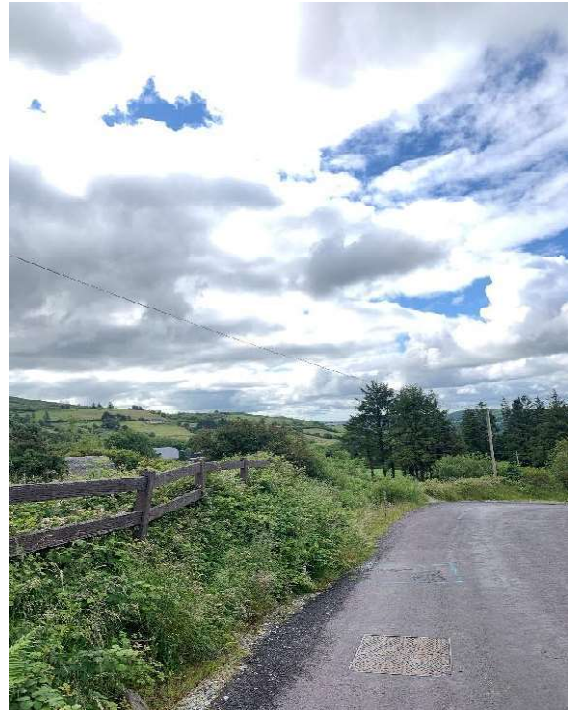
Image : 30 Joint bay on the road here with a links box and communications chambers visible.
