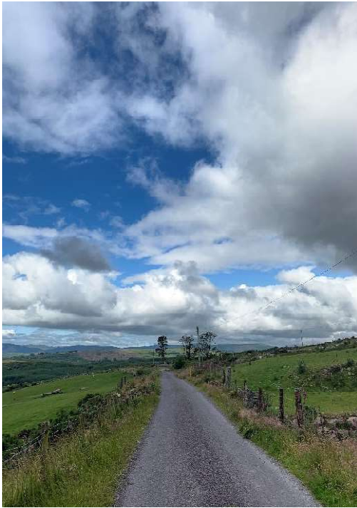
Image : 27 Esb cable maker visible on the RHS of the road edge.
