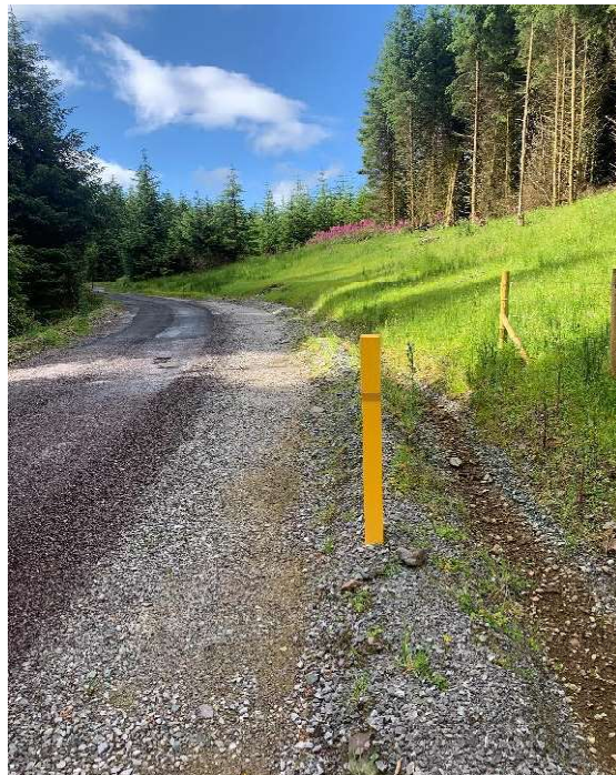
Image : 15 Ebs marker post pictured along road edge before another possible joint bay location
