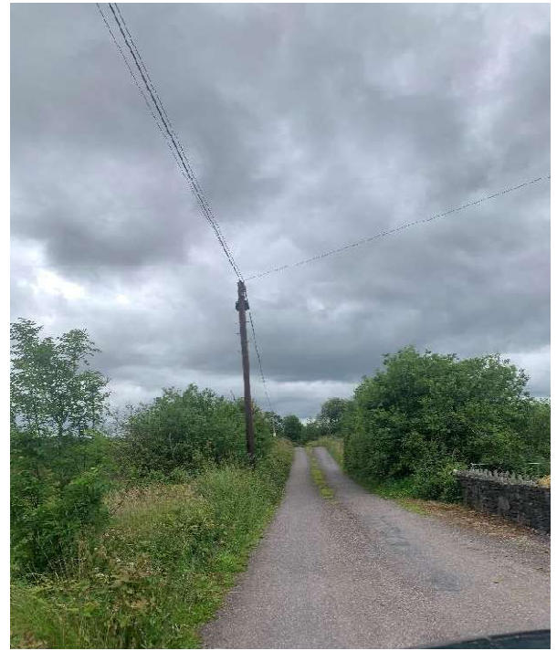
Image : 63 Storm pipe crossing road at stone wall parapet
