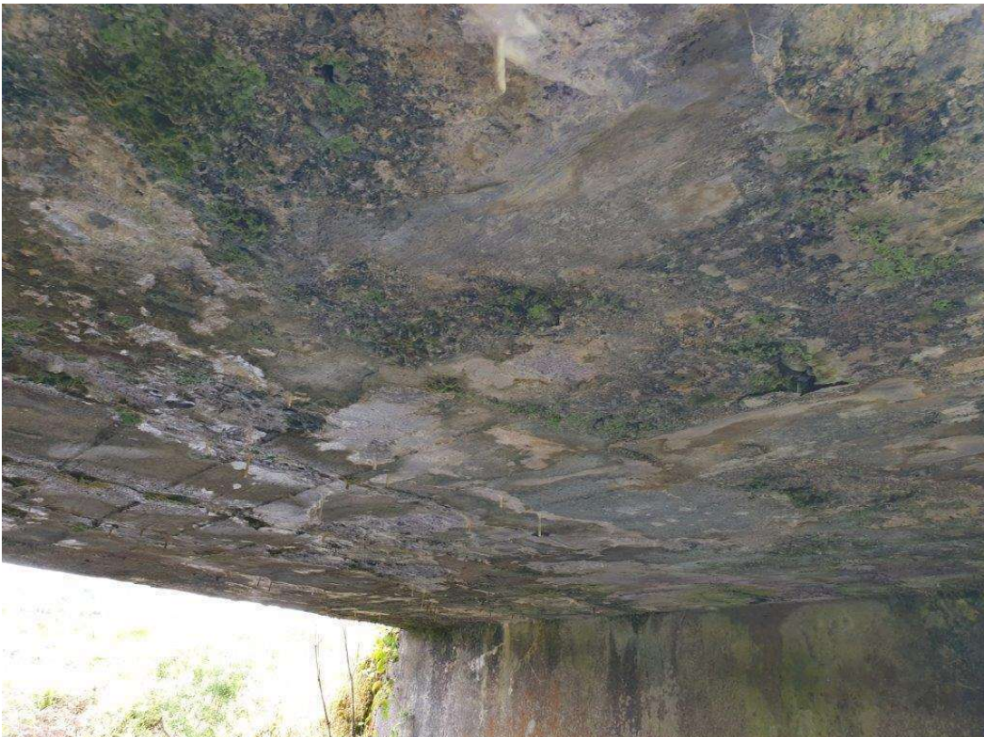
General view of the soffit of the bridge deck showing typical condition
