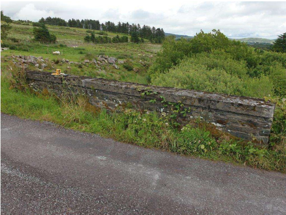
General view of the east parapet
