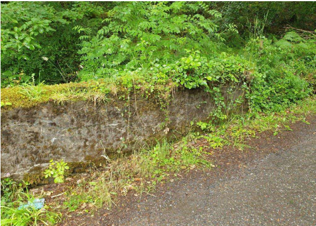
General view of the north verge and parapet
