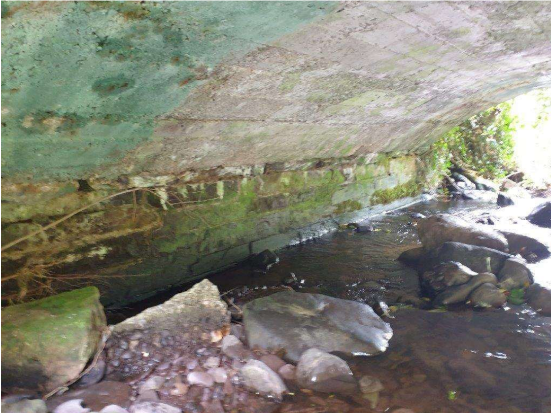
Typical condition of abutment & arch barrel
