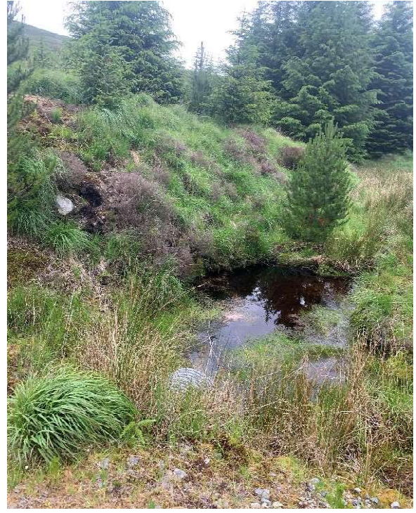
Image : 79 Twin wall UPVC storm pipe crossing under road
