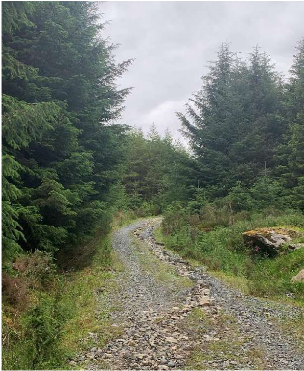
Image : 72 Forestry track on Coillte lands very step and heavily rutted
