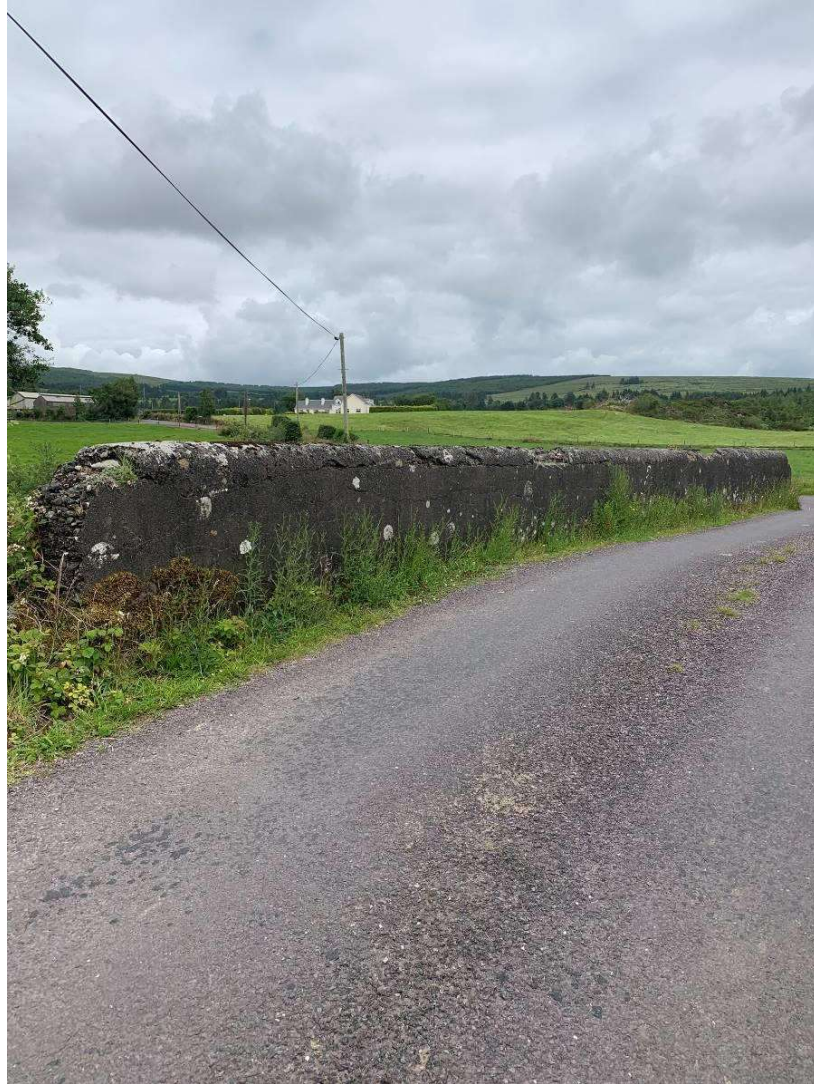
General view of the bridge parapet
