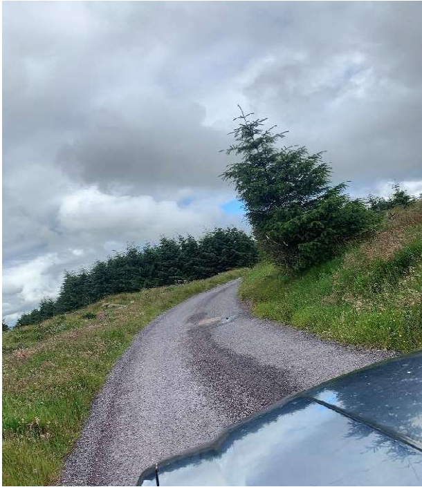
Image : 17 Joint bay located at this point
