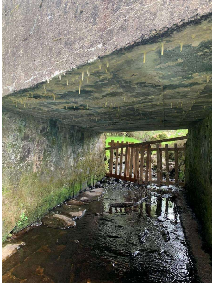
General view through the bridge showing the deck and abutments
