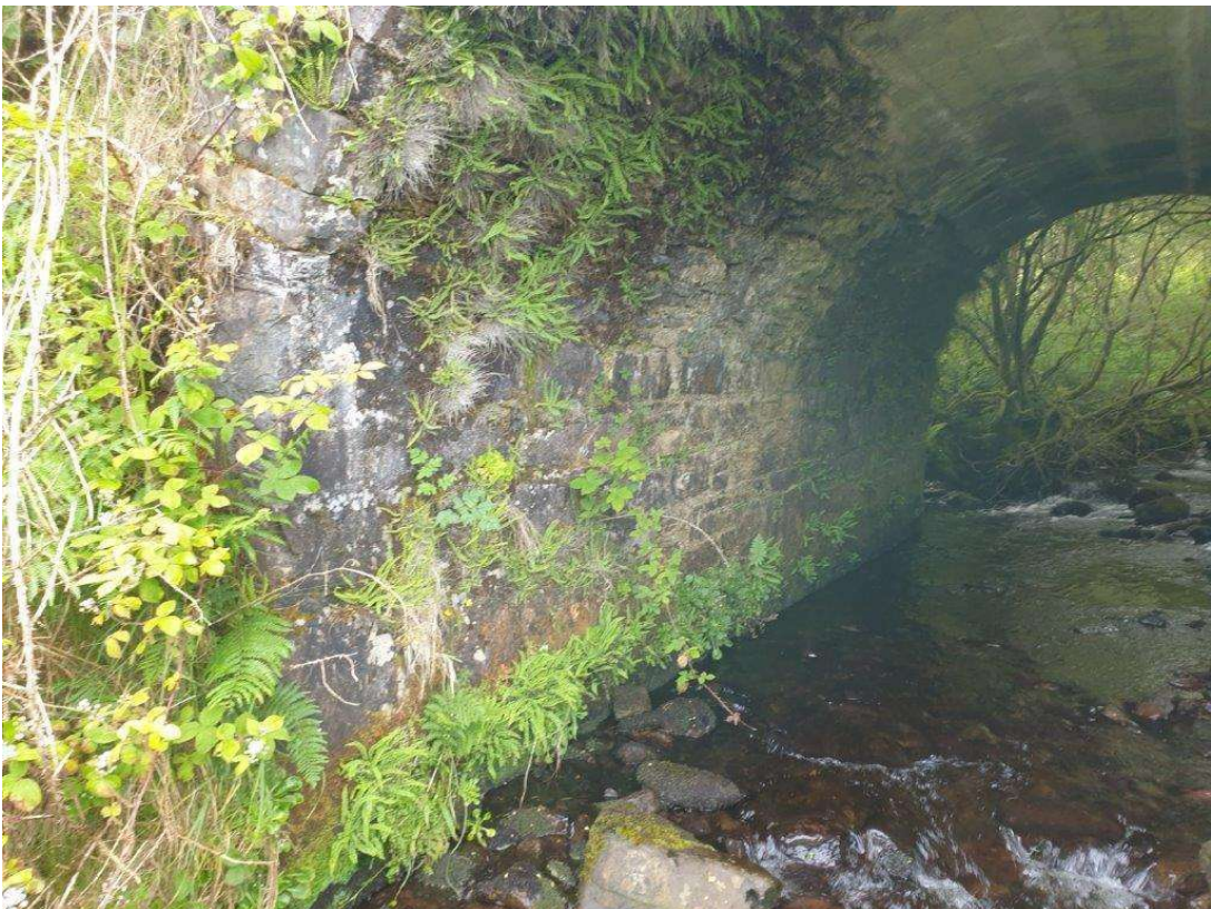
General view of the south abutment
