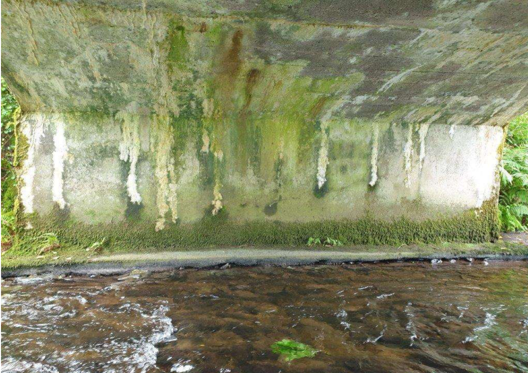
General view of the north abutment
