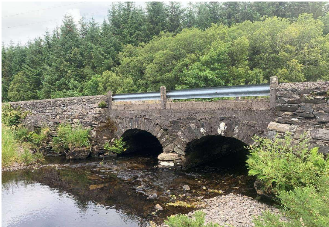
General view of bridge elevation
