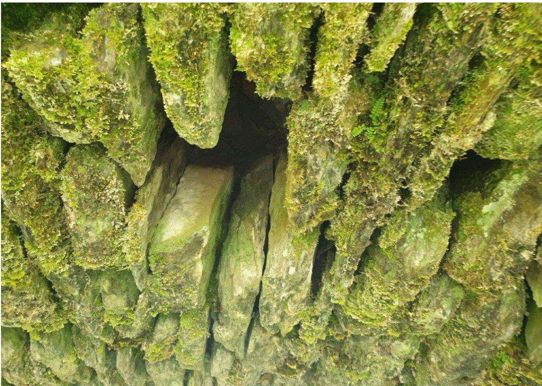
Dropped / missing stones in the arch barrel towards the north face of the bridge
