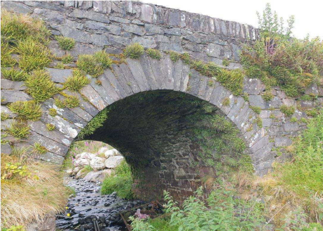
General view of the south elevation
