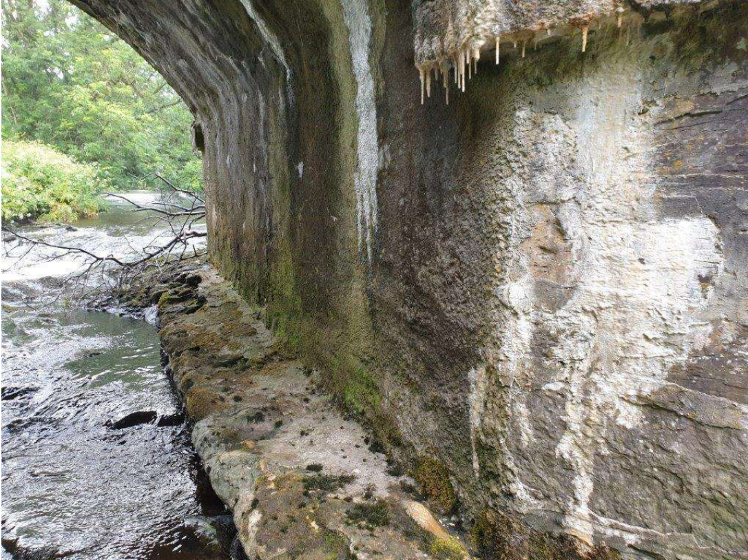
Typical pier condition
