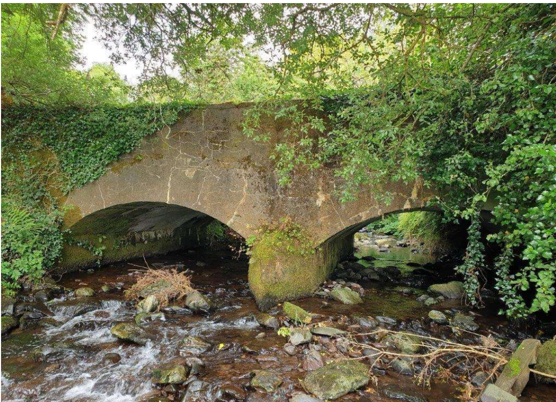
General view of south elevation
