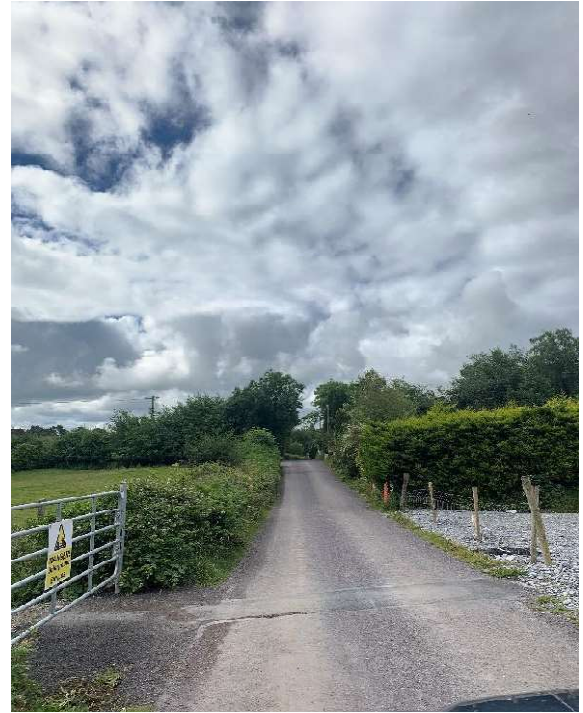
Image : 36 Visible trench scar crossing road at this location
