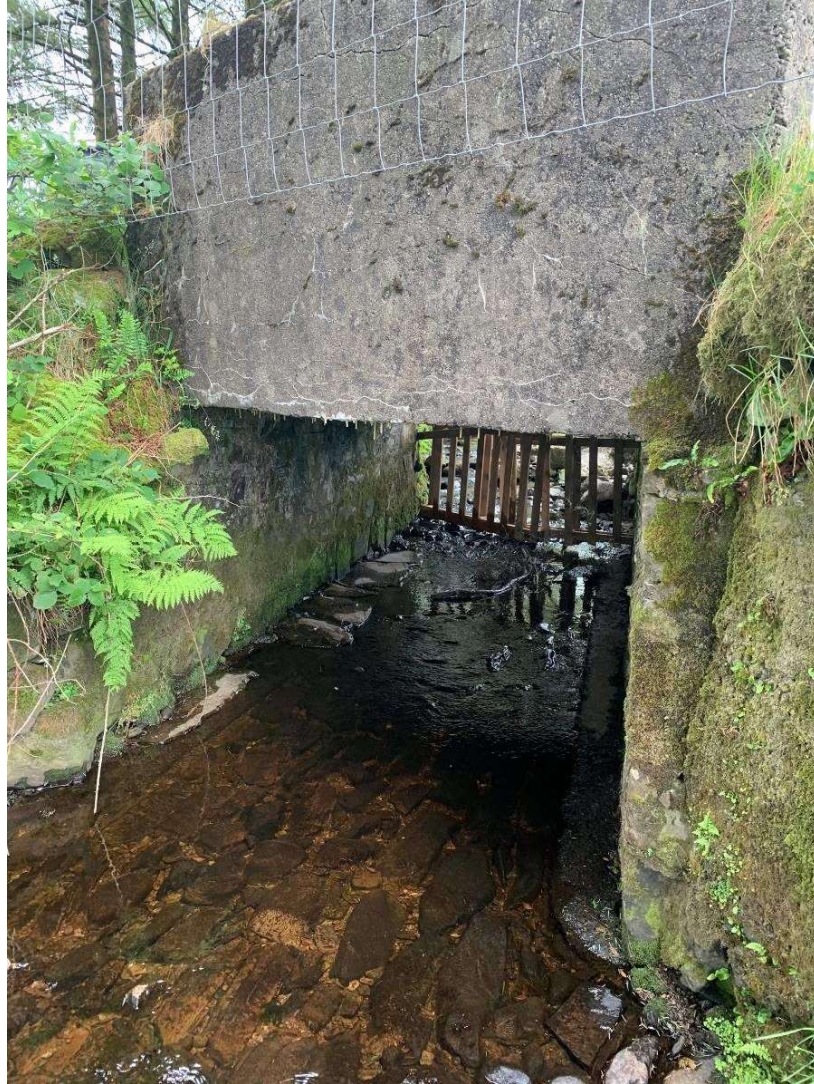
General view of the bridge elevation
