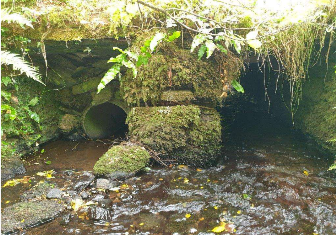
General view of the east elevation
