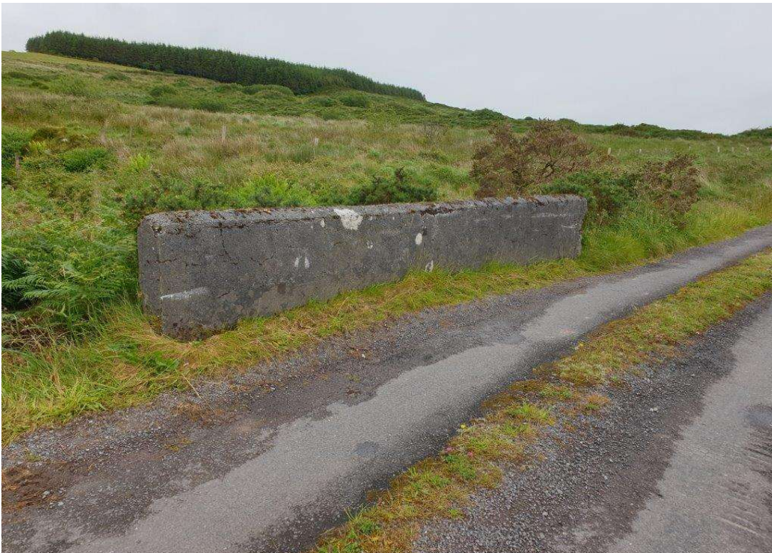
General view of bridge surface and east parapet
