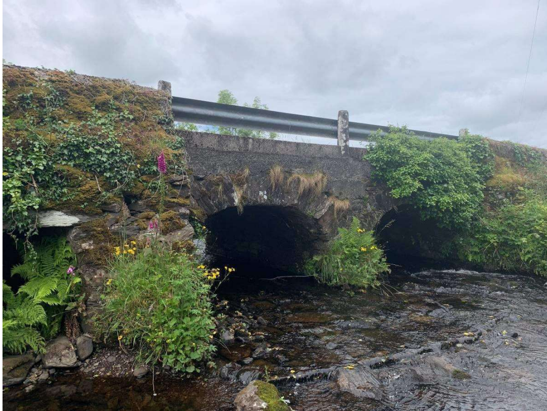
General view of bridge elevation, relief culvert shown to the left
