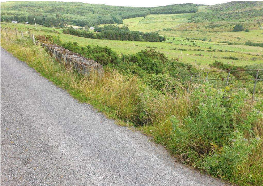
General view of the south parapet
