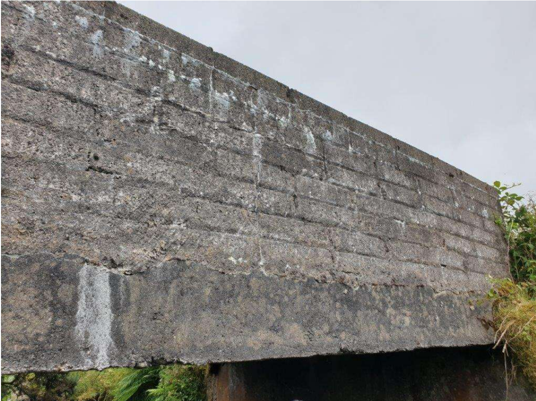
General view of the west elevation
