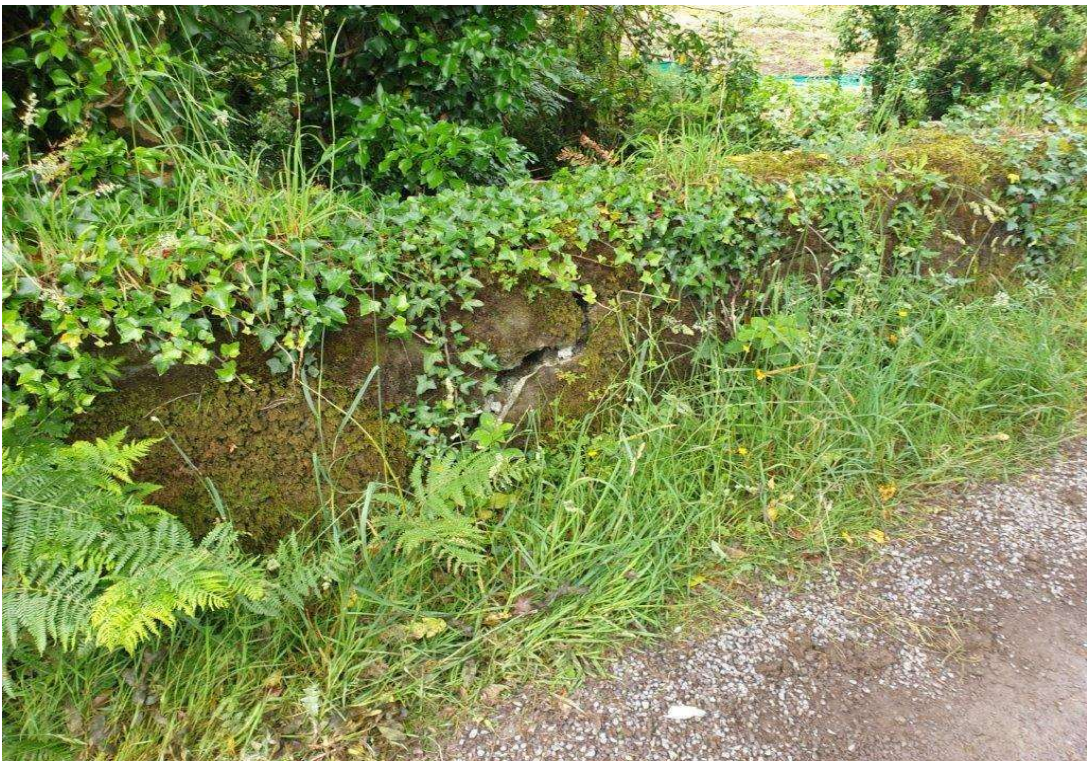
General view of the south end of the east parapet
