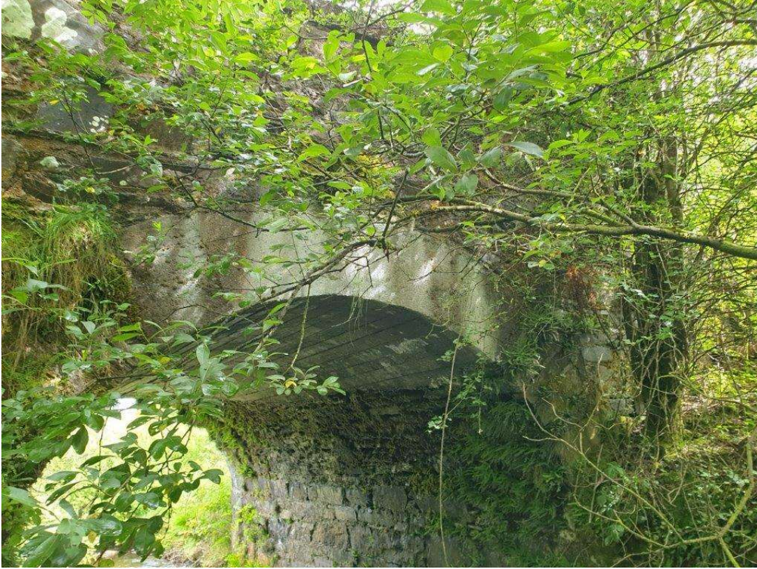
General view of the west elevation
