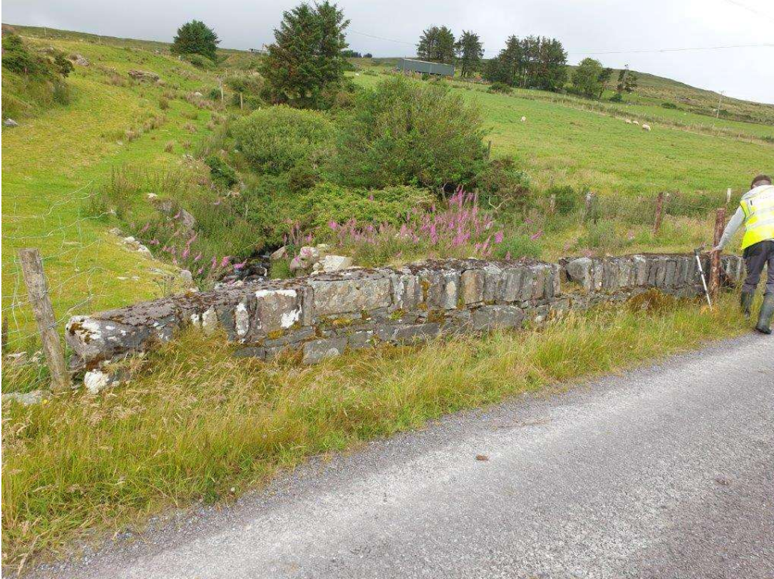
General view of the north parapet
