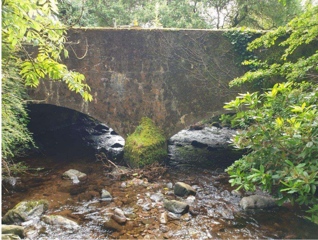
General view of the west elevation
