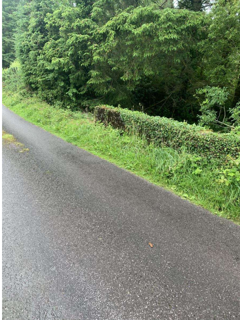
General view of the east parapet
