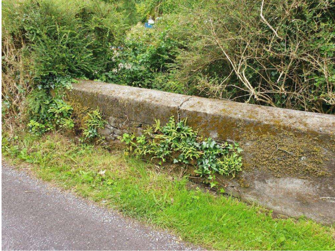
North parapet, west end
