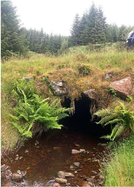
Image : 76 Box culvert crossing under road
