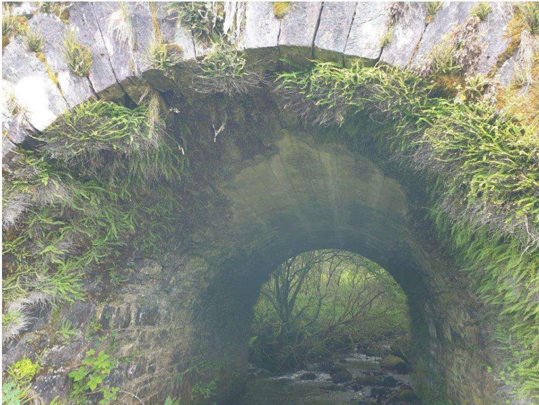
General view of the arch barrel from the east
