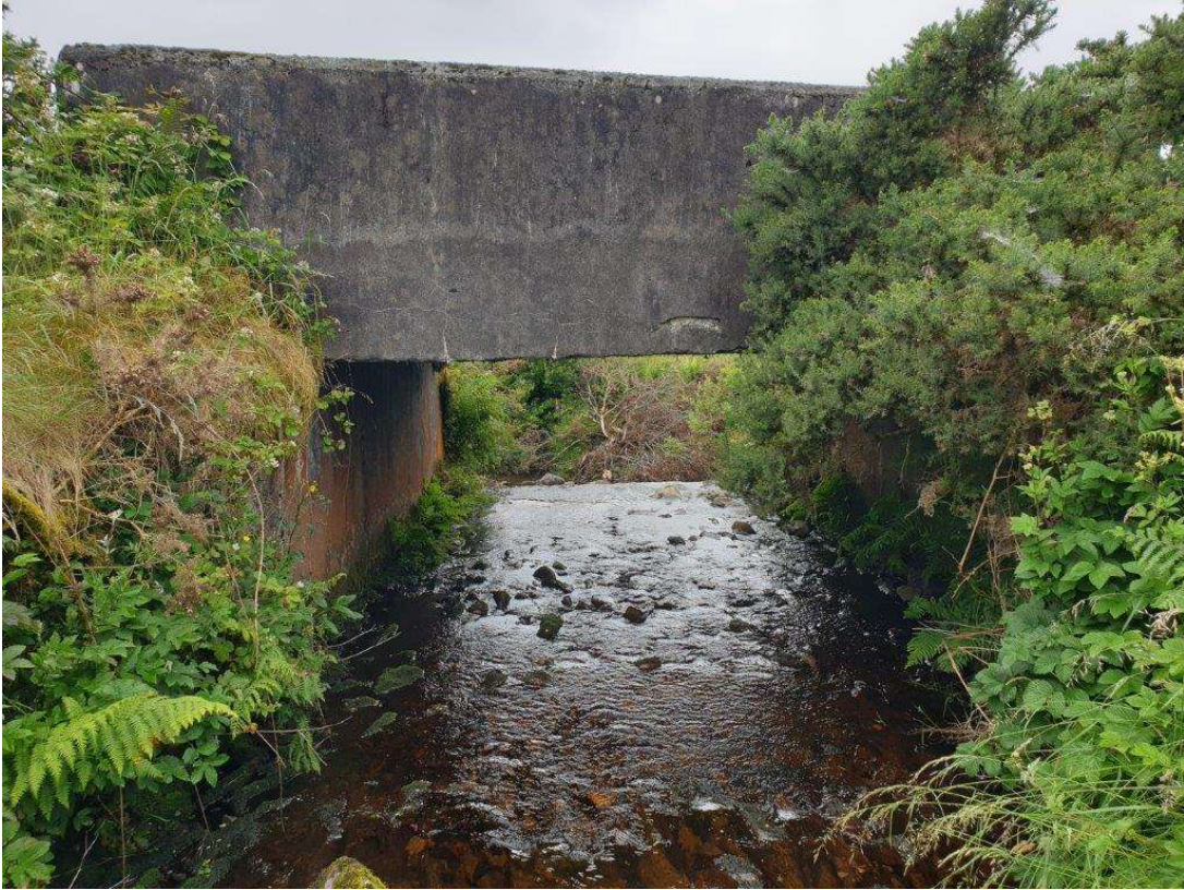
General view of east elevation, looking downstream
