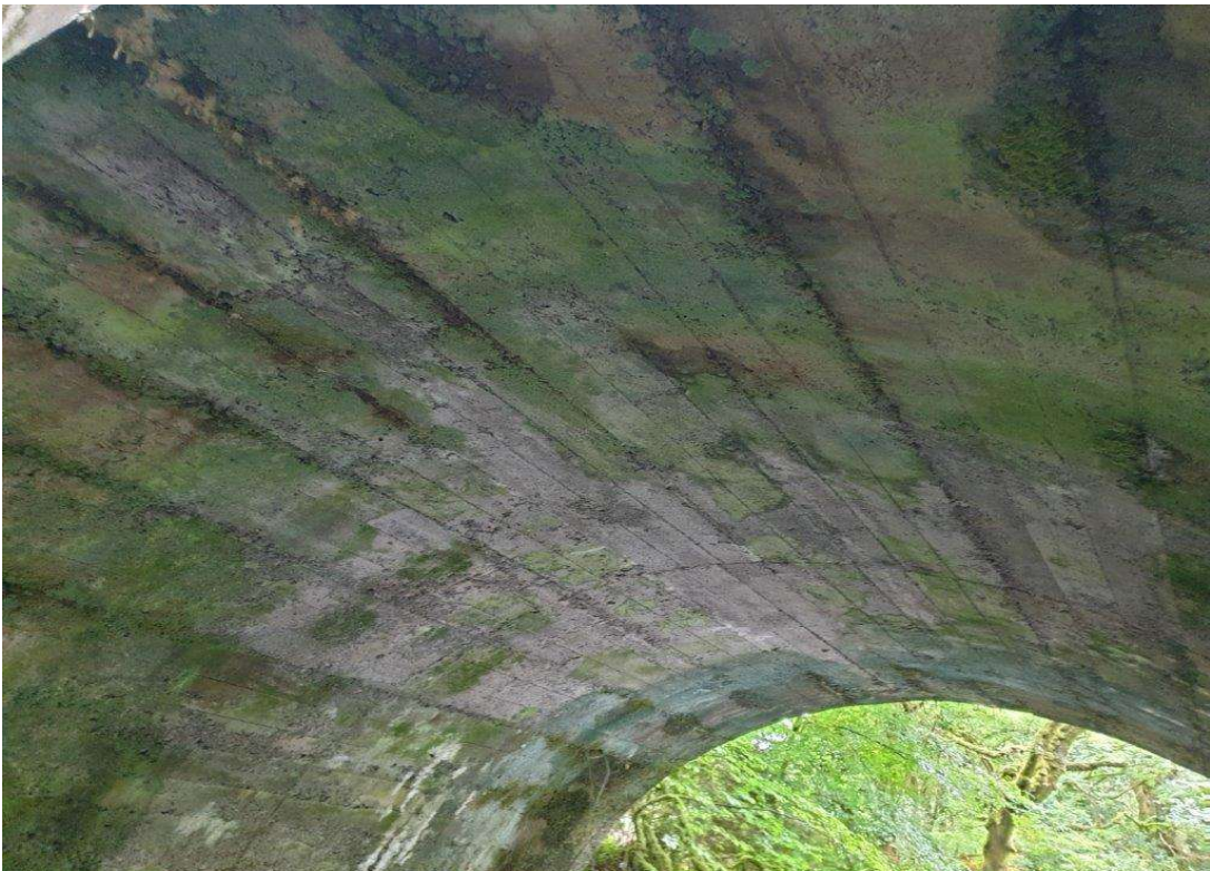
General view of the arch soffit
