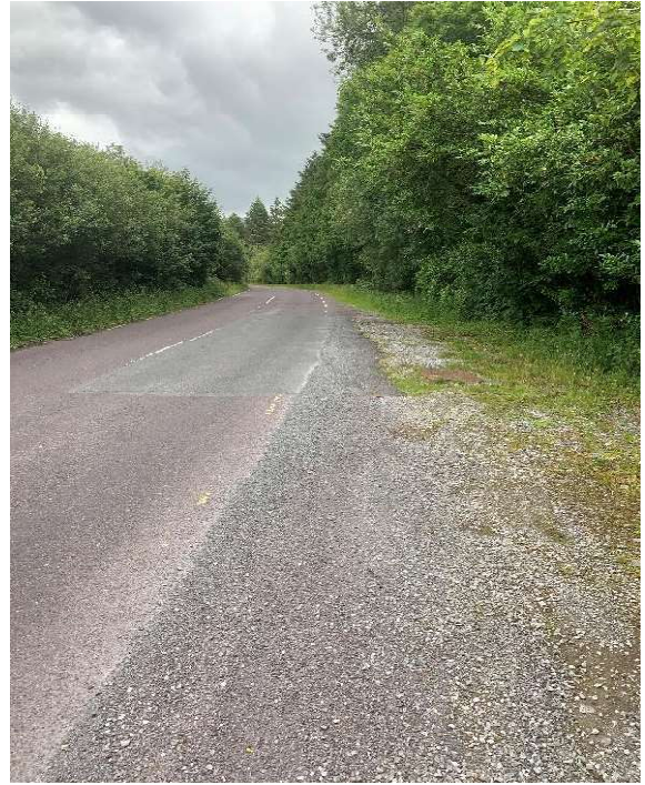
Image : 42 Joint bay on the road here with a links box and communications chambers visible.
