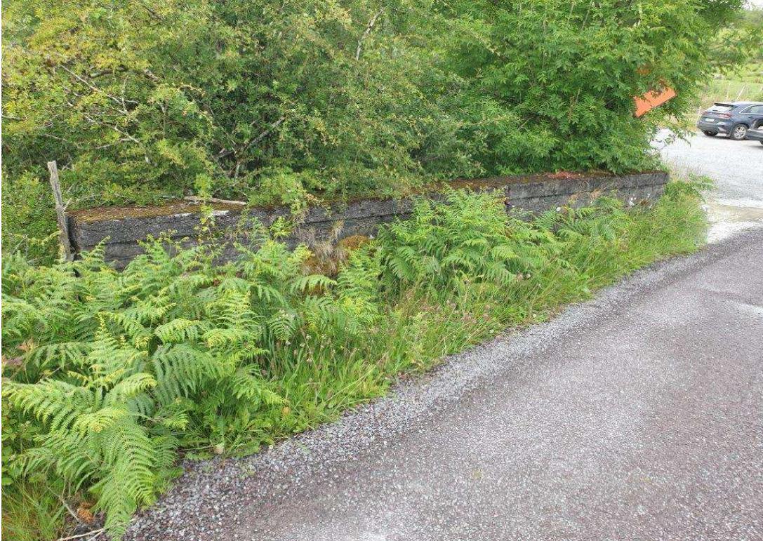
General view of the west parapet
