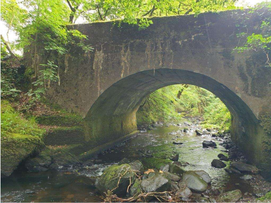
General view of the north elevation, looking downstream
