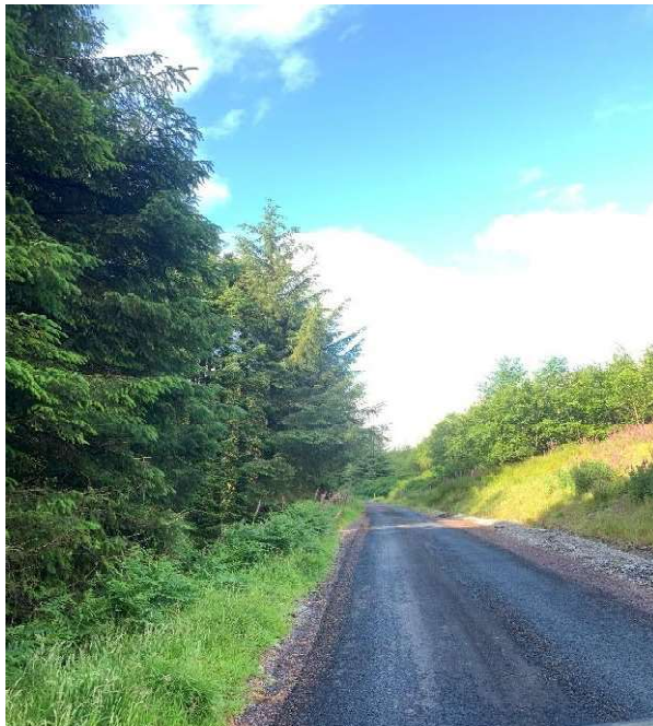
Image : 11 Possible joint bay location of existing cable running in the road
