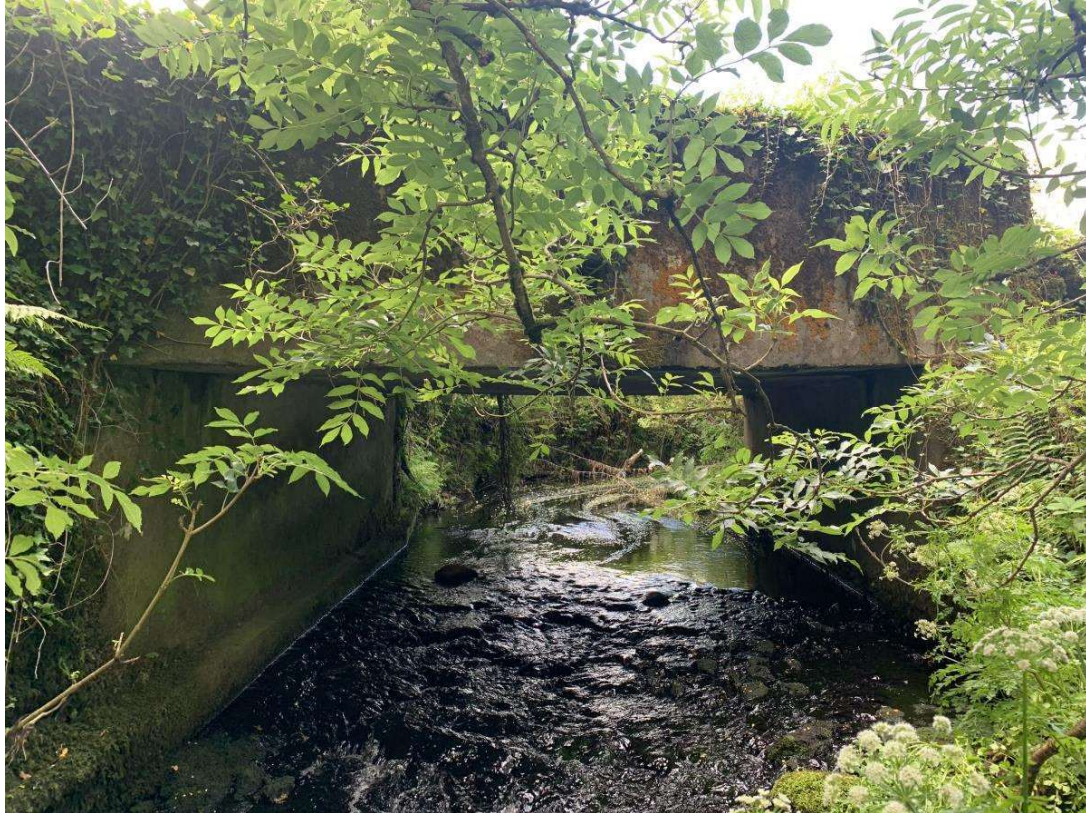
General view of the bridge elevation
