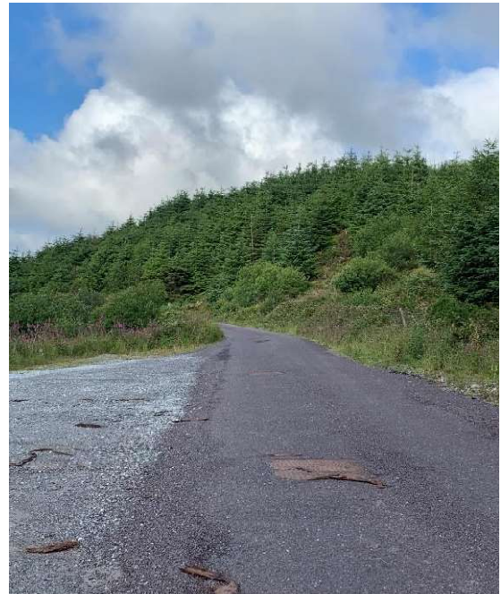
Image : 12 Joint bay on the road here with a links box and communications chambers visible.
