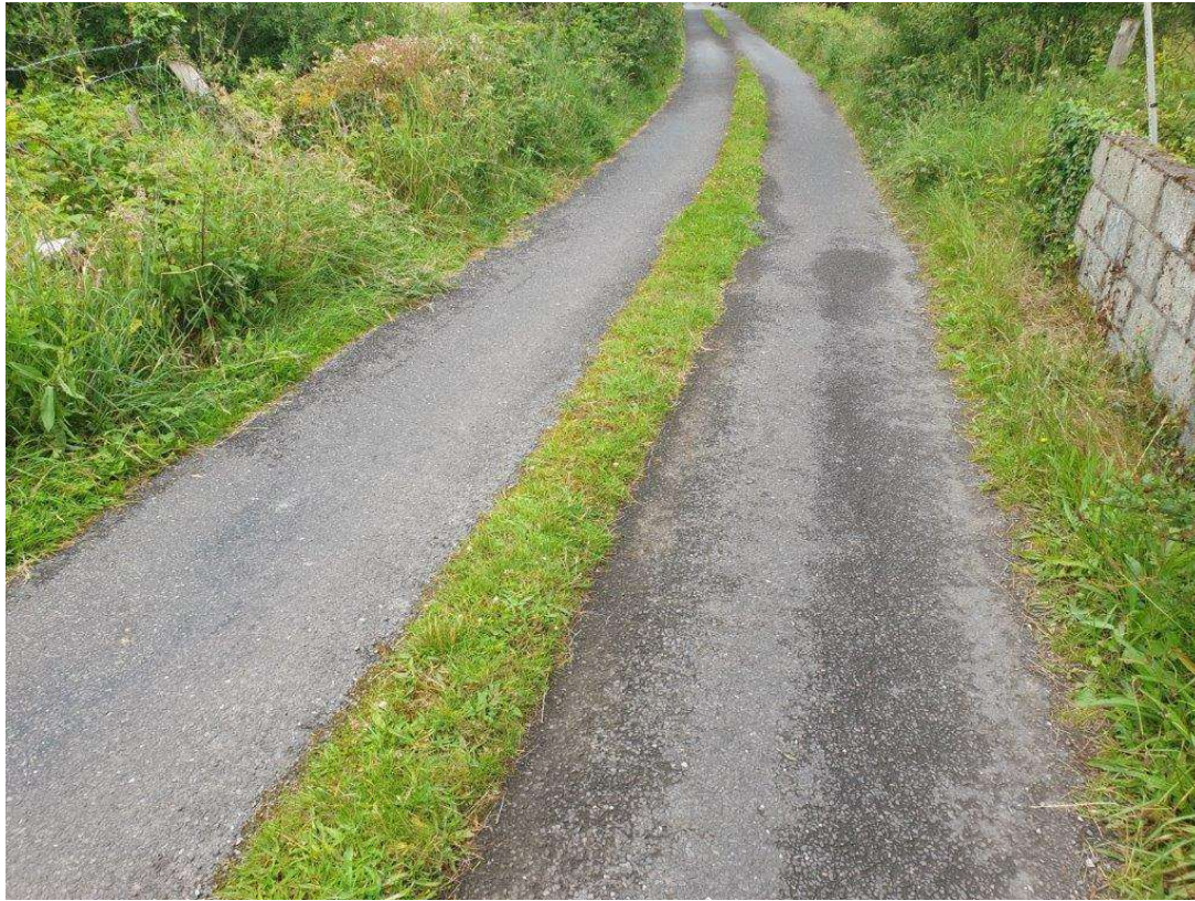
General view of bridge surface
