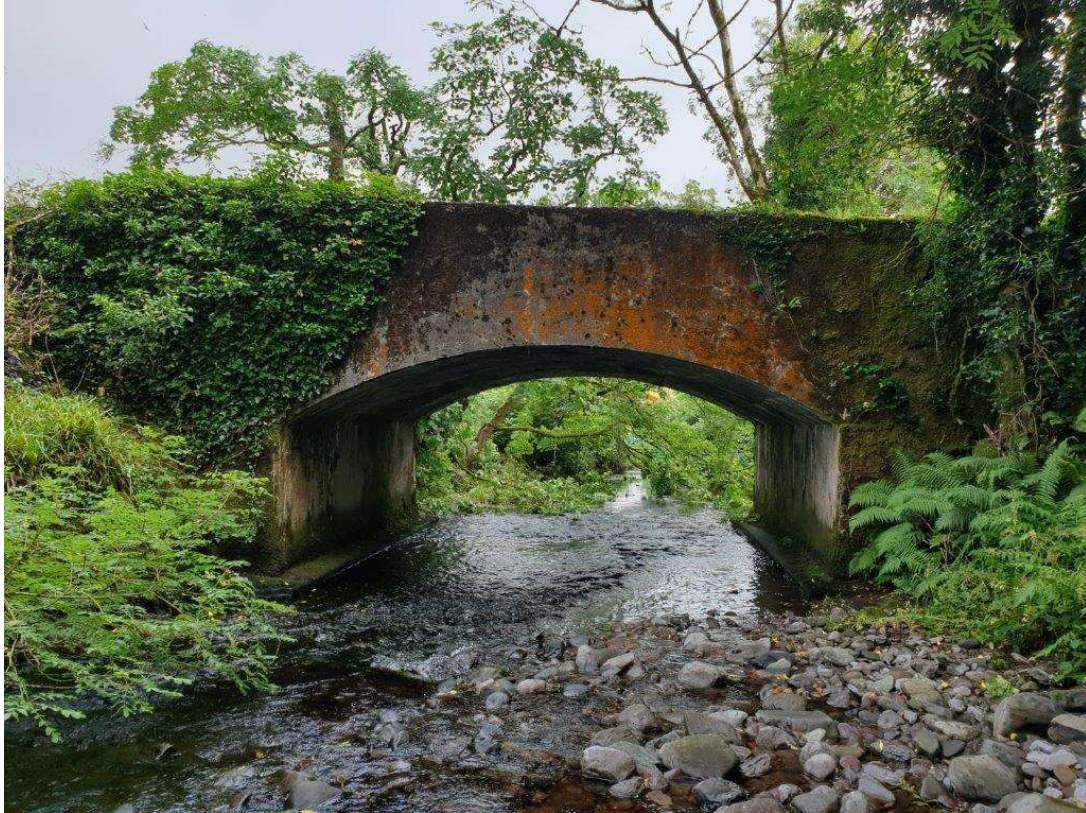
General view of the west elevation, looking downstream
