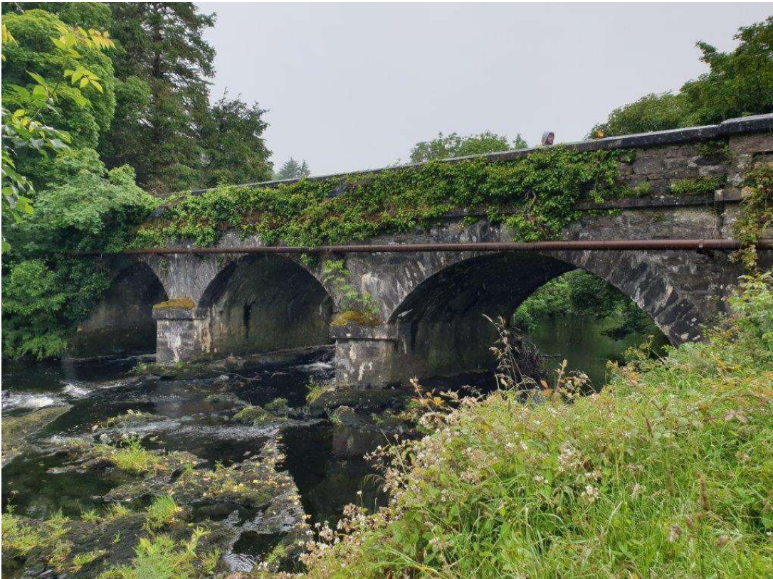
General view of the south elevation
