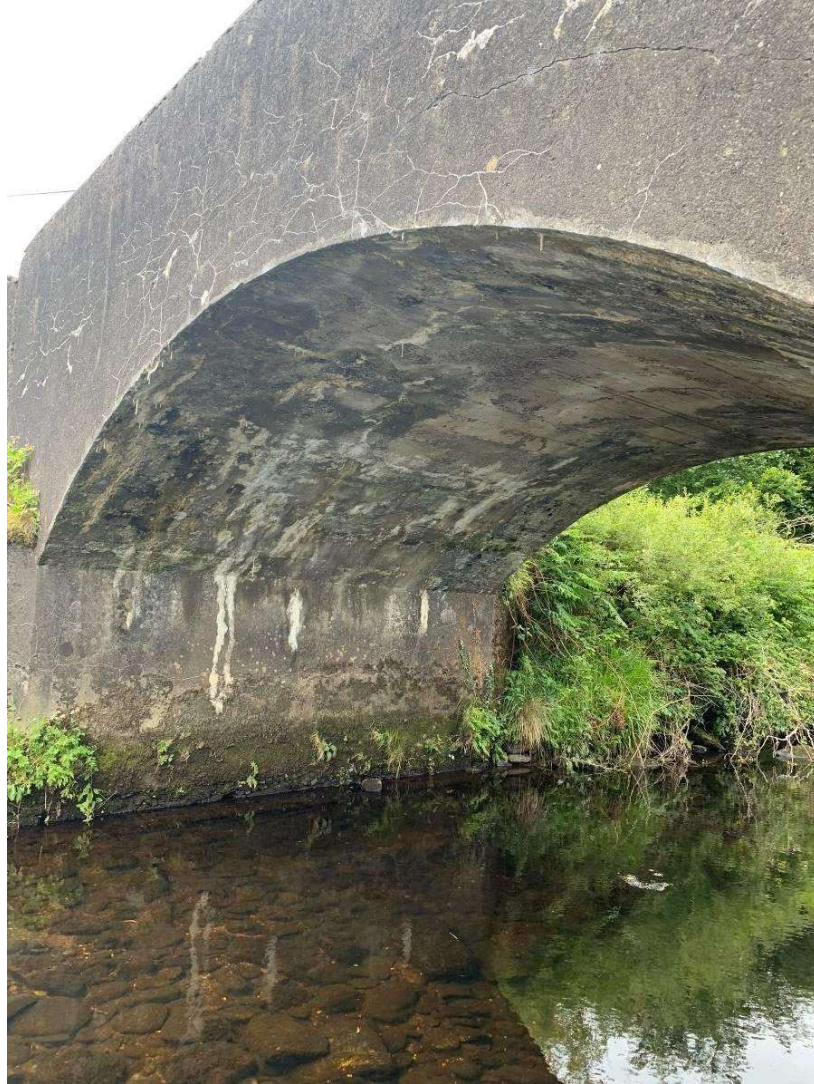
General view of bridge span showing typical condition of arch barrel and abutment
