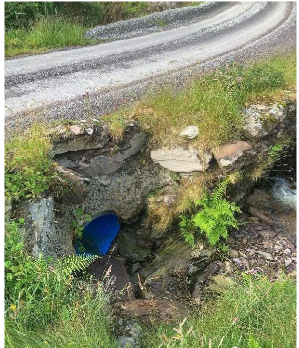
Image : 14 Two twin wall drainage pipes crossing under road. Depth of cover approx. 500mm
