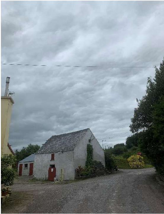
Image : 68 Farm house and out buildings in close proximity just before you cross the N22
