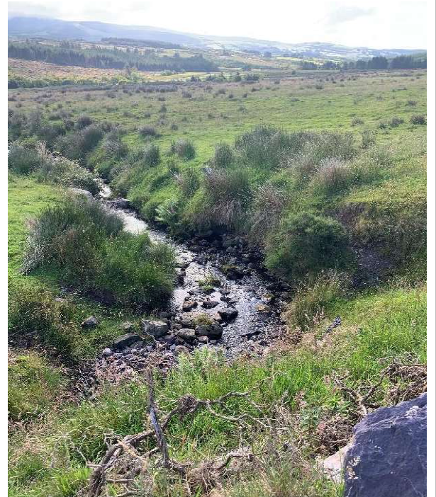
Image : 6 Stream crossing under road at this point
