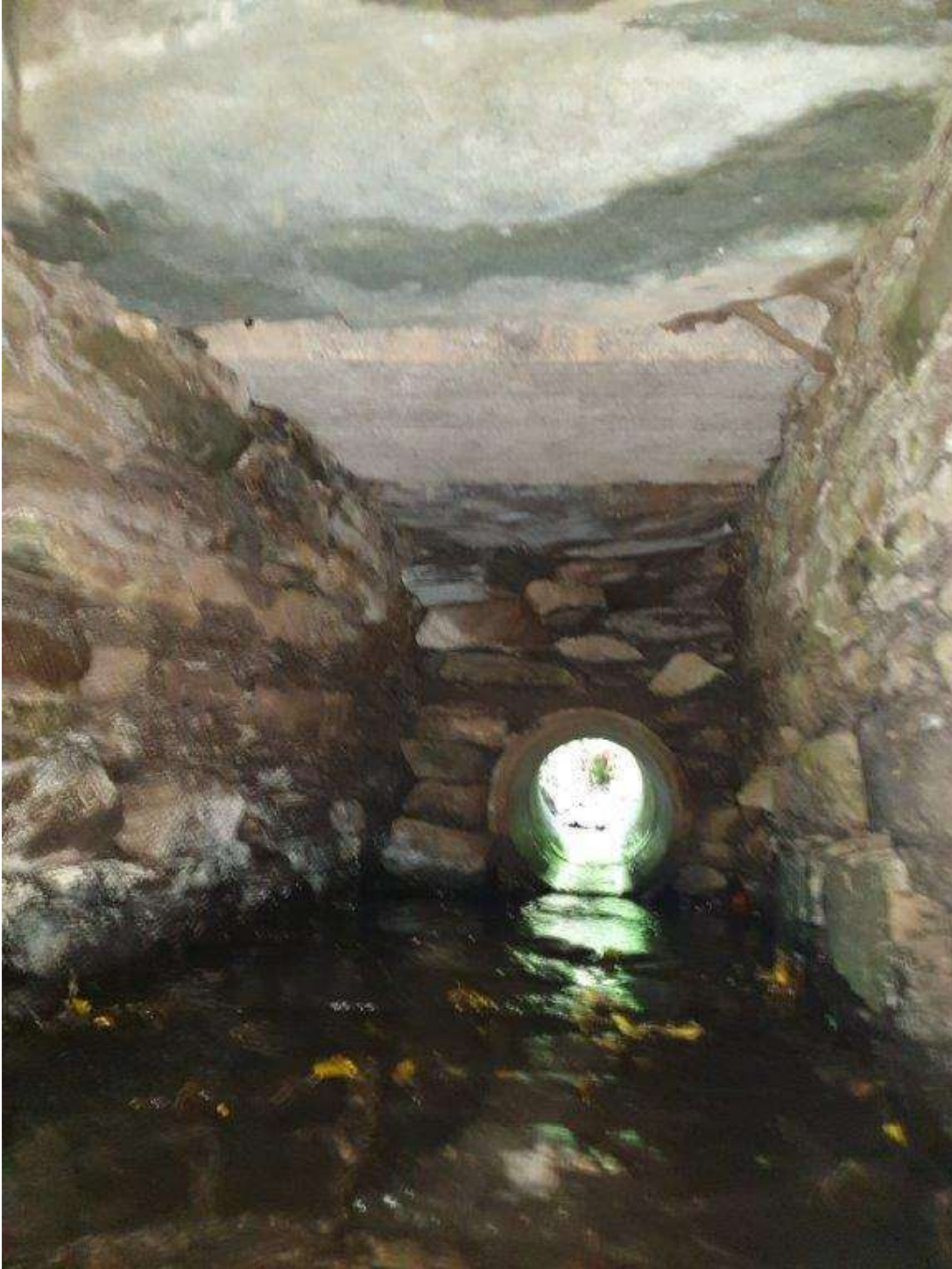
View of south span from the west
