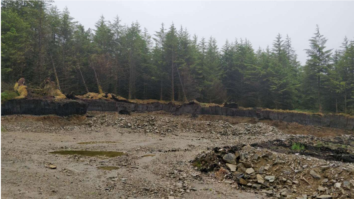
Figure 6-3: Ground conditions observed along route C
