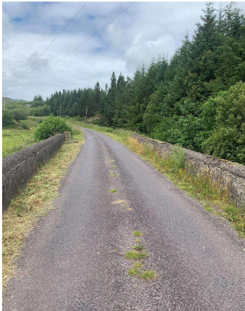
General view of the bridge surface
