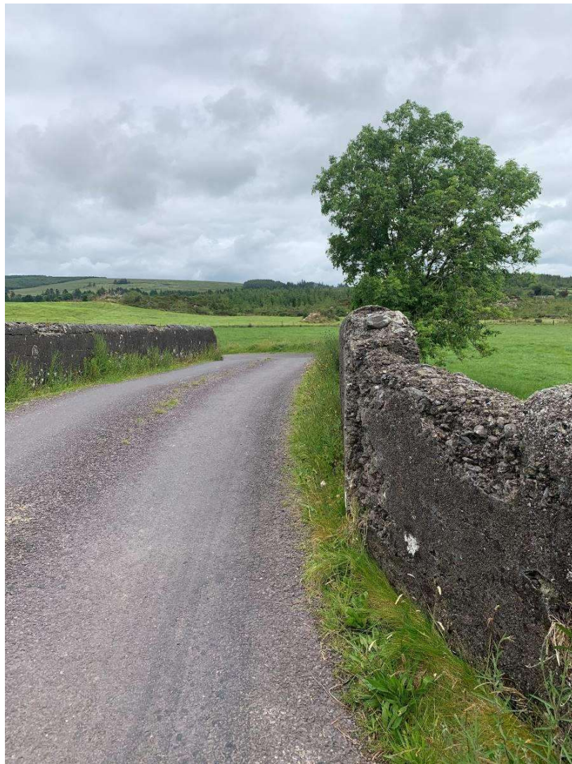
General view of the bridge surface
