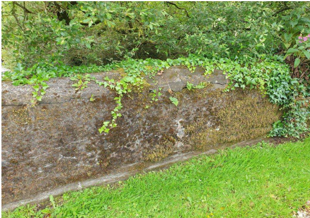
South parapet, east end
